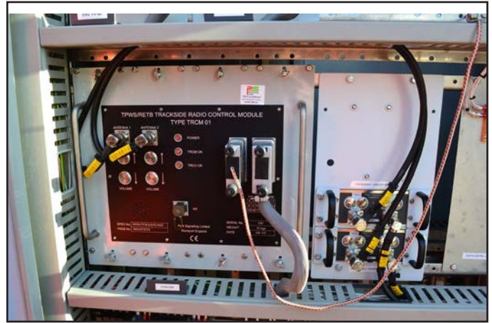
Figure 13 – Trackside Radio Control Module (TRCM)
